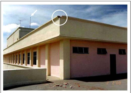
The above picture shows the damaged concrete roof corner (circled) caused by a direct lightning strike. This college building was installed with an unconventional air terminal (arrowed). Debris from such damages is a hazard to people and cars who may be loitering just below the corner at the time of the incident. More than 80% of buildings in Kuala Lumpur that have been installed with the un-conventional air terminals have at least one of this lightning strike damage features on them.
