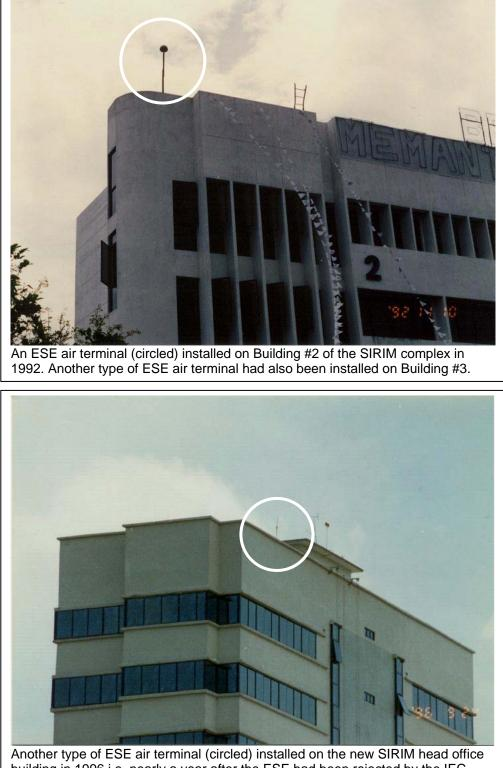
Another type of ESE air terminal (circled) installed on the new SIRIM head office building in 1996 i.e. nearly a year after the ESE had been rejected by the IEC. This building was struck and slightly damaged by lightning not long after this picture was taken.
