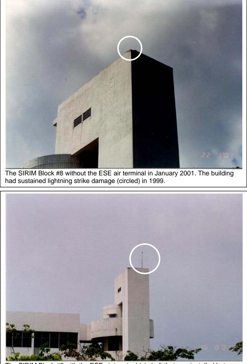
The SIRIM Block #8 with the ESE air terminal (circled) that was installed between January and August 2001. SIRIM still continued to install the ESE air terminals even though the ESE technology had just been dropped from the new Malaysian standard.
