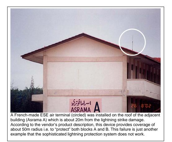
The Subang Jaya school complex of about half a dozen buildings was installed with three lightning attracting air terminals that is claimed to have protection coverage of about 50 m
