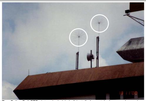
Two Spline Ball CTS air terminals (circled) installed on a telephone exchange in Kuala Lumpur. The failure of these terminals have also been reported in scientific papers.
