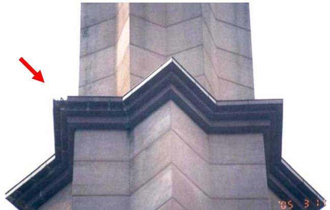
Fig. 7: Close-up view of the lightning damaged section of the minaret (arrowed).
