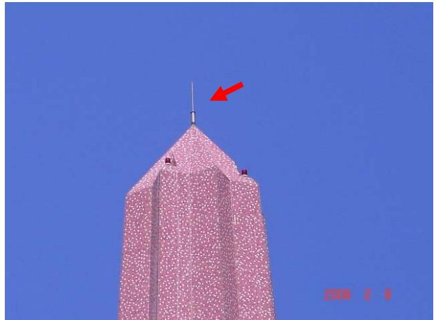
Fig. 6: An ESE air terminal on the apex of the minaret (arrowed).
