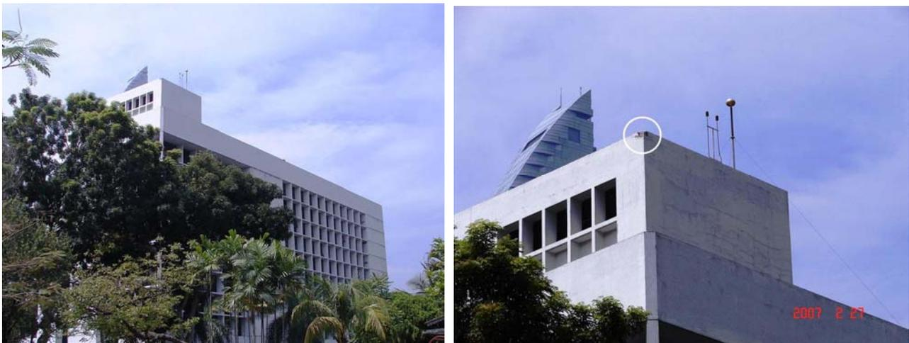
Fig. 2 – A bypass occurred close to a CVM air terminal that is positioned according to the proprietary collection volume method.
