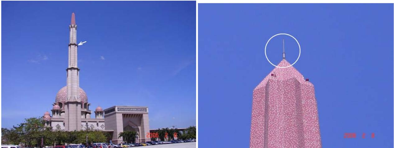
Fig. 7 – The picture on the left shows the Putrajaya mosque and the position of the bypass (arrowed). The picture on the right is a close-up photo of the apex of the minaret and shows the ESE air terminal.
