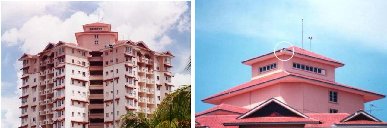
Fig. 1 – A bypass occurred close to an ESE air terminal that is manufactured and positioned according to the NFC 17-102 standard.
